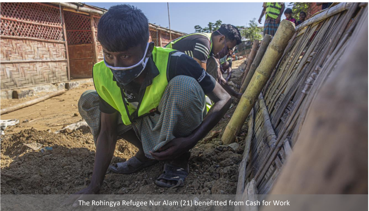
Slope stabilization using bamboo and geo bags
